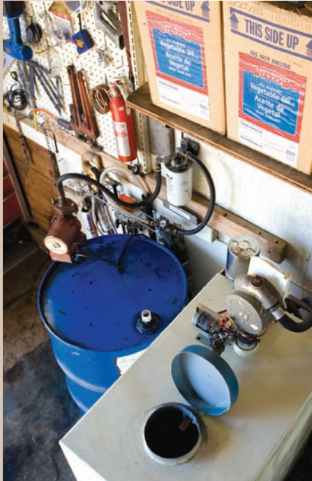
Rempen built his own low-tech filter system, shown here, using old blue jeans and a 55-gallon drum.
